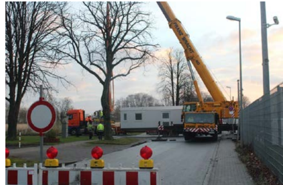
Transport and preparing installation
