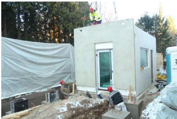
Assembly of the sandwich panels on site
