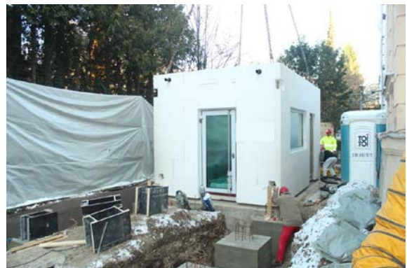
Off-loading and installation on site
