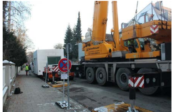
Transport and preparing installation
