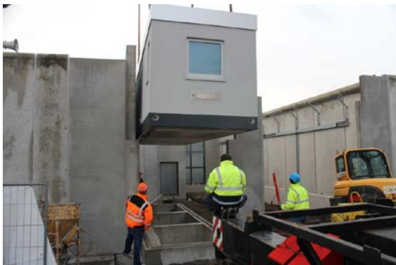
Off loading and installation on site
