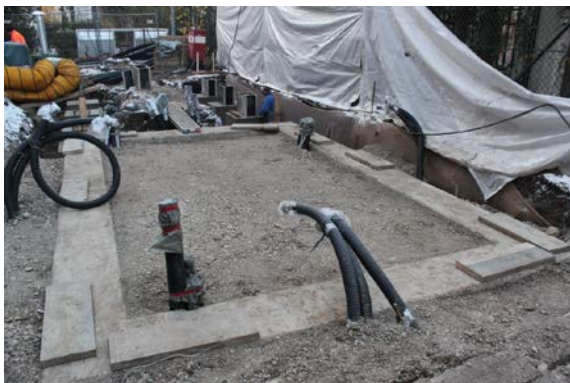
Preparation of the pre-constructed concrete base
