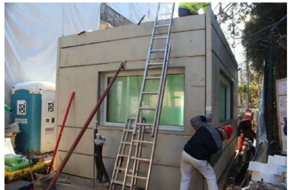
Assembly of the sandwich panels on site
